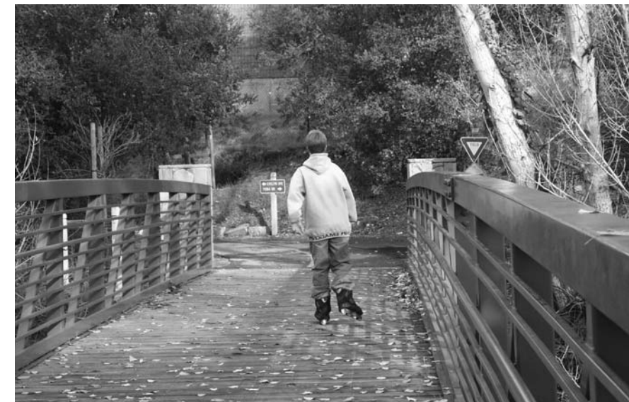
Pedestrian Bridge over Stevens Creek Photo courtesy of Davis Fields
